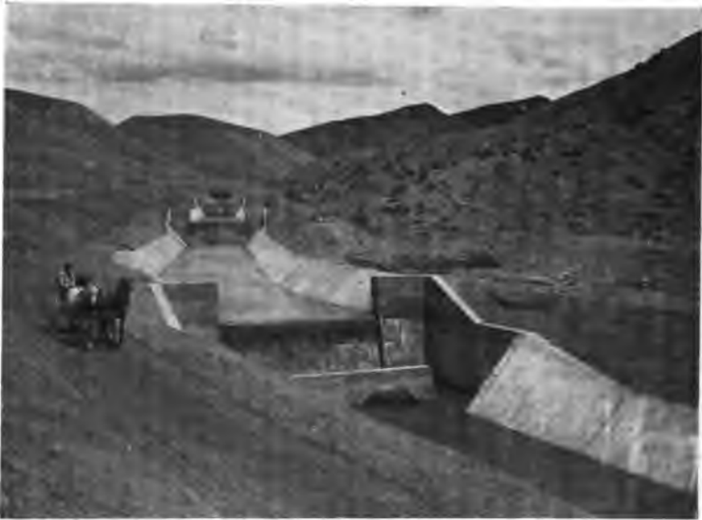
FIG. 127.—Series of Concrete Drops on South Canal, Uncompahgre Valley, Colorado.
